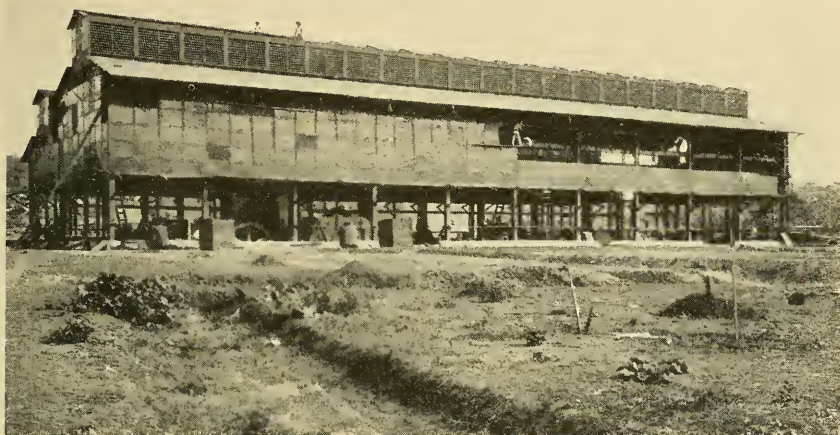
THE PUMPING STATION AT PLATO
